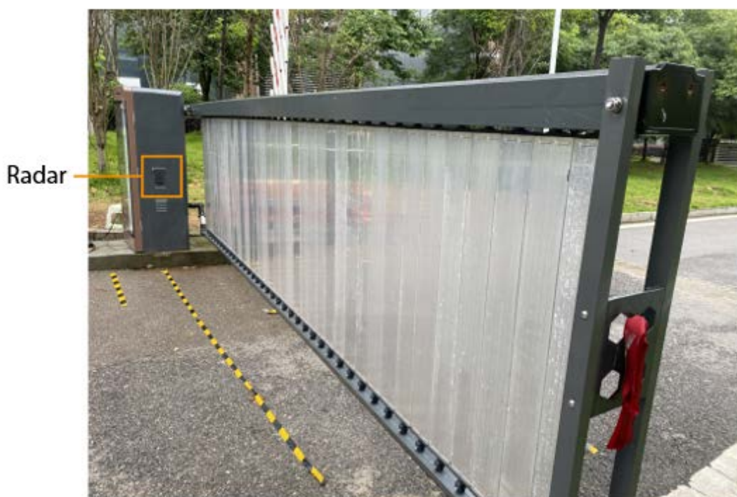
Figure 3-4 Radar installation completed
